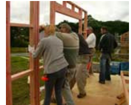
The wall goes up!
